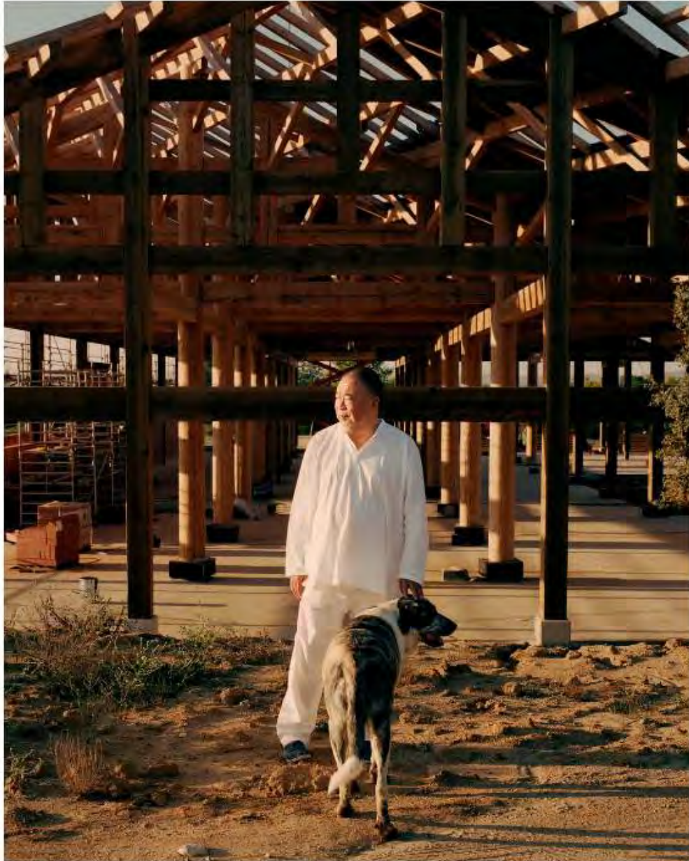
Ai's new 30,000-square-foot studio, on a perch close to his home, is a near copy of his studio in Shanghai, which Chinese authorities demolished upon its completion. Based on traditional Chinese architecture, the frame is made from timber, the roof from clay tiles and the floor from stone. Jo Metson Scott
